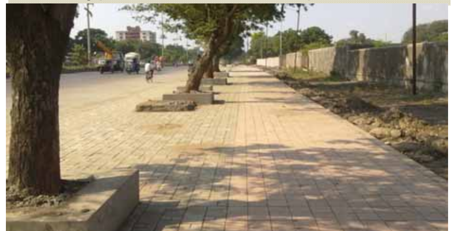
Trees retained along Footpath
