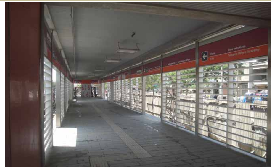
Prototype Bus Station Completed
