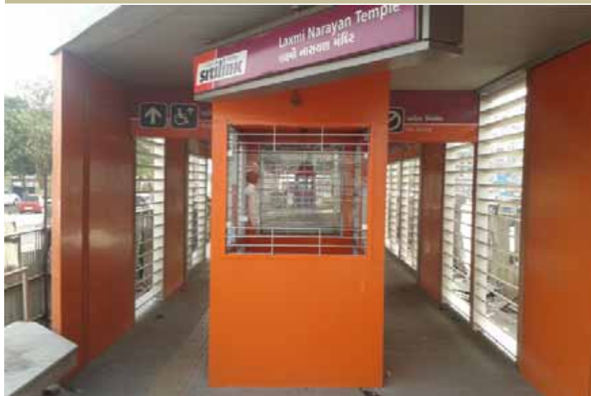
Prototype Bus Station Completed
